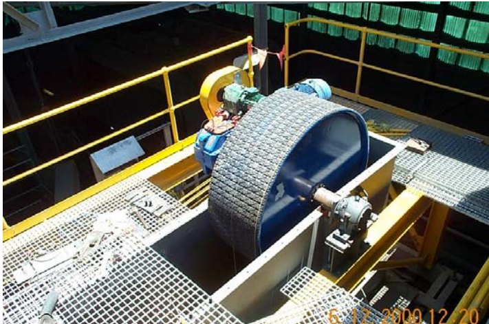
The head lagging is shown during installation of the belt.
